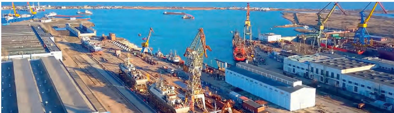
A panoramic view of the Zaliv shipyard facilities. On the right-hand side of the photo is one of the largest shipbuilding docks in Europe: at 364 metres long and 60 metres wide, it has no equivalents in the RF. It is there that in May 2020, the construction of the two helicopter-carrying amphibious assault ships, Sevastopol and Vladivostok, for the Black Sea Fleet of the RF is scheduled to begin. The photo from the BlackSeaNews archive, February 2020
